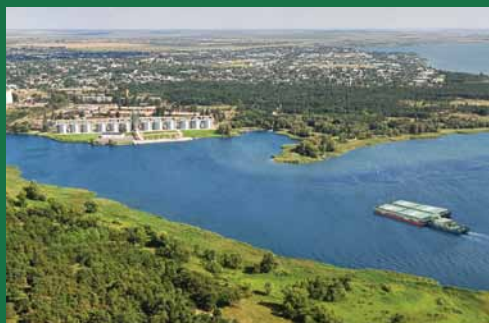
Kamianka-Dniprovska River Terminal before the destruction of the reservoir [289]
