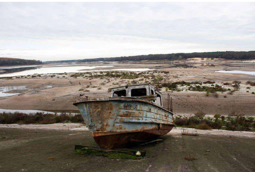
Bottom of Oskil River Reservoir (multipurpose facility including small HPP) severely damaged during the battle for Kharkiv in 2022. by Mariia Solodovnyk, Suspilne Ukraine JSC
