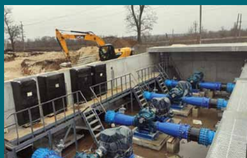
Construction of the water pipeline and installation of chambers for the maintenance, inspection, and control of the pipeline network.
